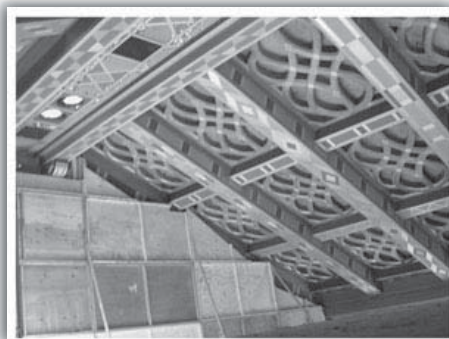
Hand-painted designs on the Main Sanctuary ceiling
